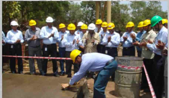
Hazardous waste Storage platform
