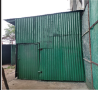
Shed made from scrap corrugated sheets
