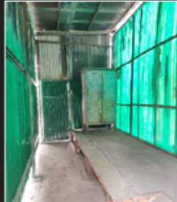
Base of shed Made from scrap metal plates
