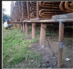
Coil bed Support from rejected pipes
